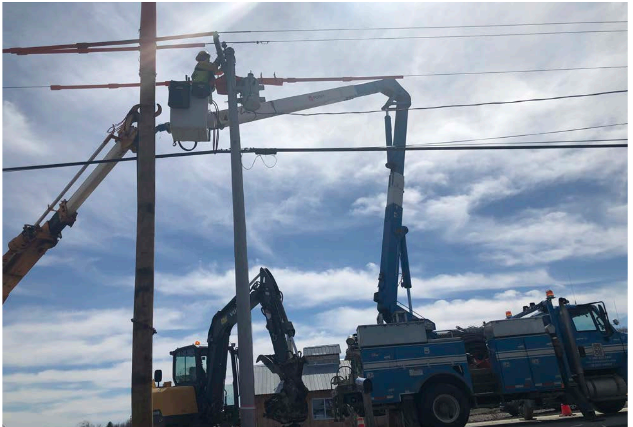
In 2019 VEC crews replaced 170 poles, including this one in Franklin.
